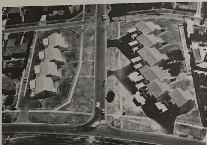
Bird's-eye view of The Turl on the left and Ripelby on the right—two further grouped housing projects developed by Garden Cities during the last few years
