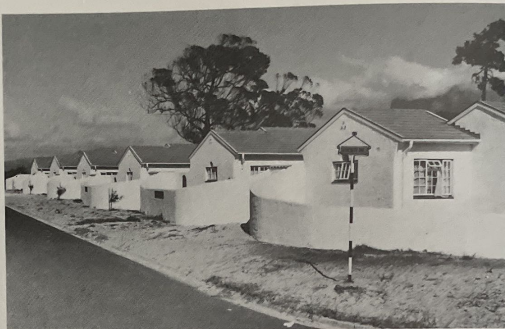
Tarragona: this photograph shows the interesting detail of the linking-walls of each unit
