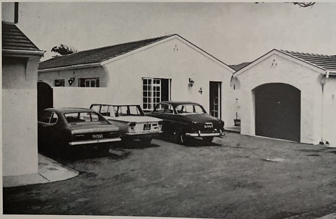
Tarragona: adequate on-site parking is essential to the concept of grouped housing—a portion of the parking space reserved for each unit
