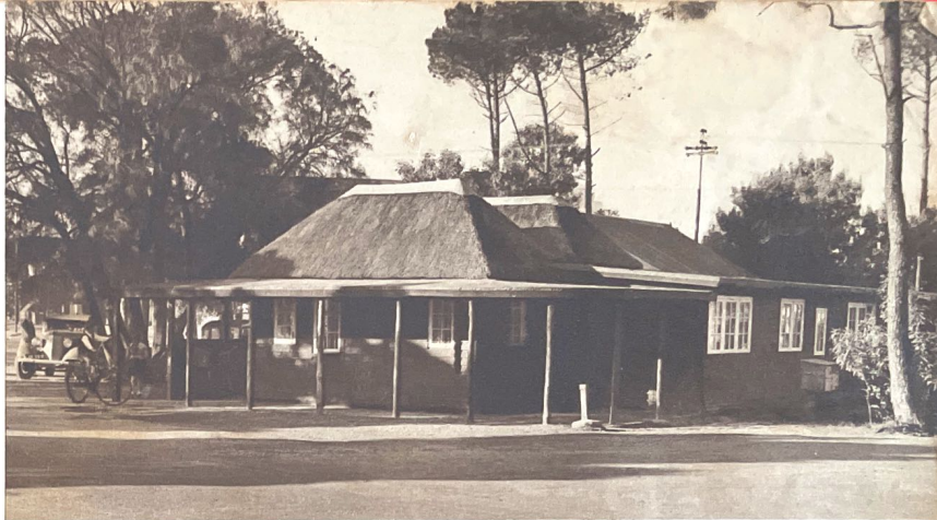
Where it all began. The original Estate Office of Pinelands still survives, though it has long been replaced by something far more ambitious.
