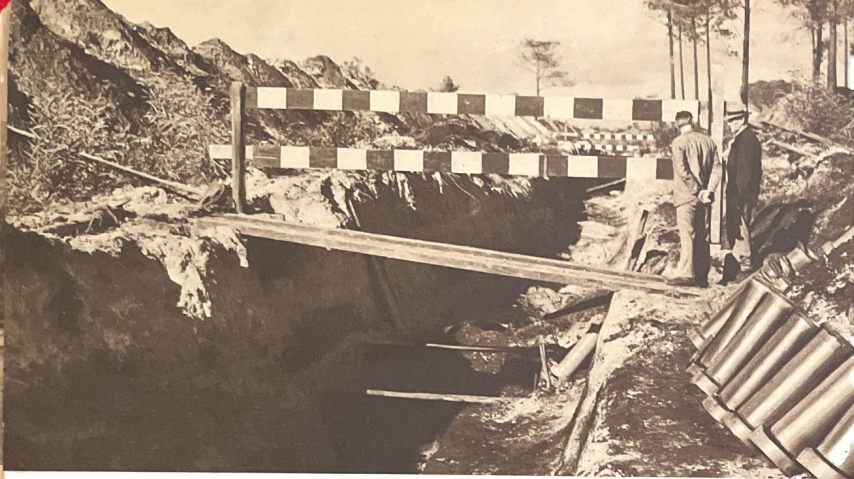
Planning for future growth at Pinelands. Laying drainage pipes.
