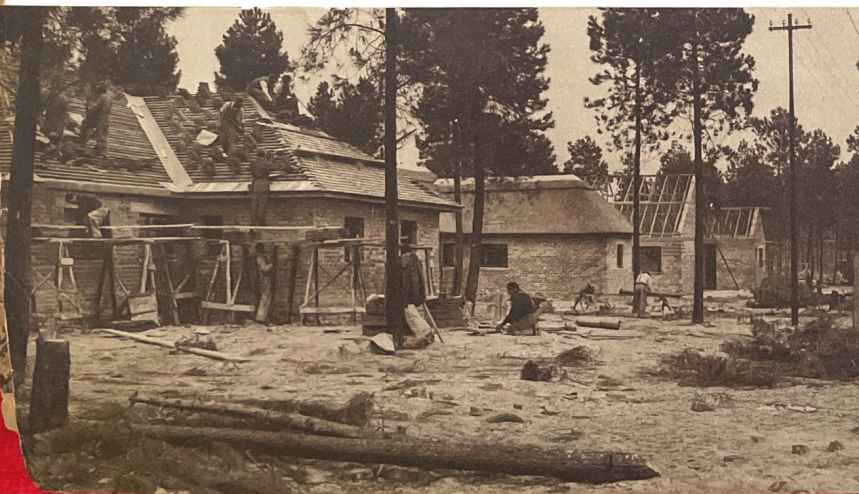
Some of the hundreds of new Pinelands houses under construction.
