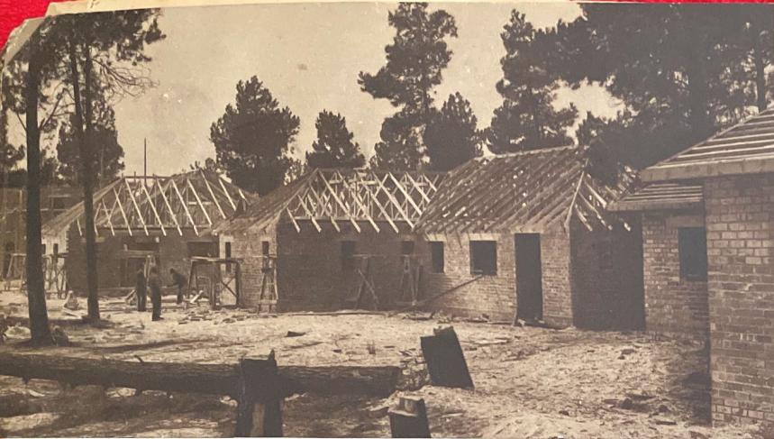
More new Pinelands houses being built.
