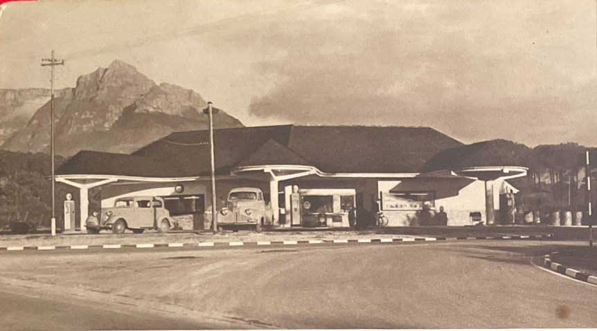
The up-to-date Filling Station operated by Garden Cities.
